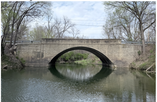
The East Fork Fishing River Bridge may be an eligible resource which was not included in the previous boundary.
