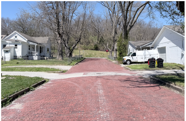
Original brick paved streets may be considered as a contributing resource to a local or national district.
